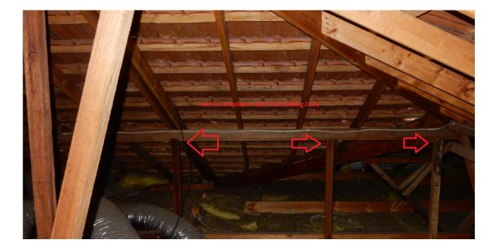
2/ Roof Void / cuts used to for the struts are not compliance the building code to support the under purling.
