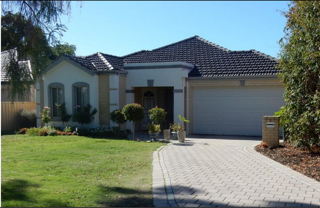
Front Elevation of the Inspected Property
